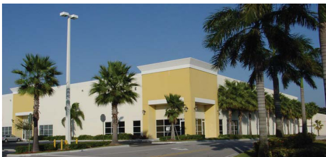
Seneca Industrial Park
