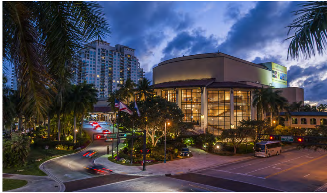
▲ Photo courtesy of the Broward Center for the Performing Arts. 47,585-square-foot Lauderhill Performing Arts Center and Library. Broward County
